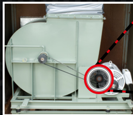
Plant HVAC System Compressor
