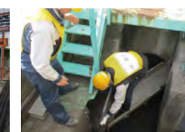
Installing cover for agricultural water inlet
