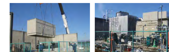
Installation of the high-efficiency power generator
